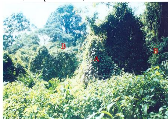
Photo-1: Neglected shrine
