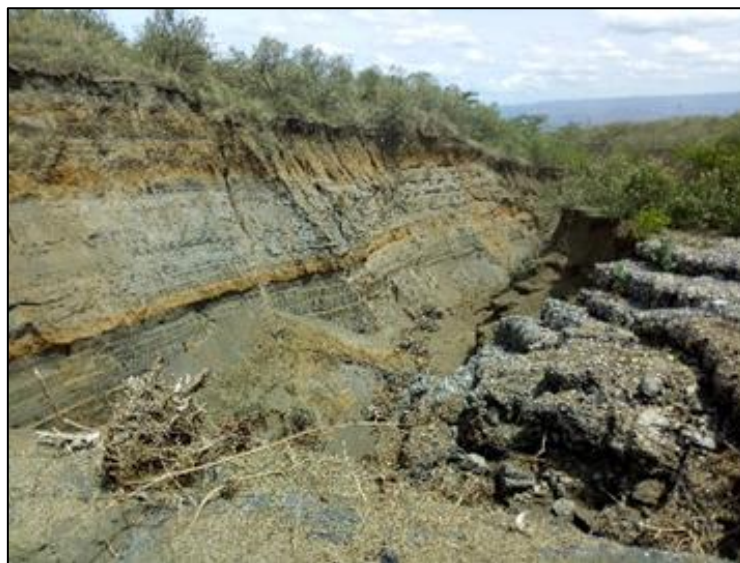
Figure 3: Gully in RAPland village
