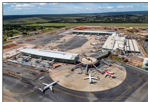
Figure 5 BSB: passenger terminals. Source: Infraero, 2019.
