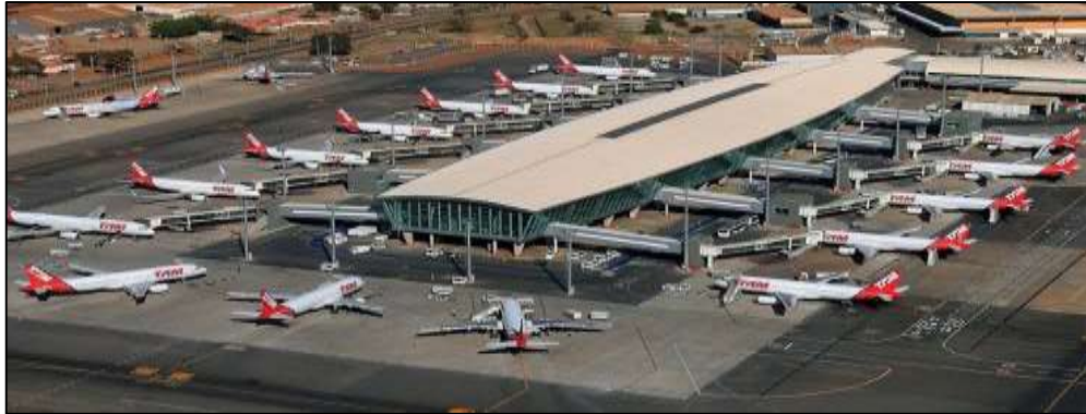
Figure 2 BSB International Airport. Source: Infraero, 2019.
