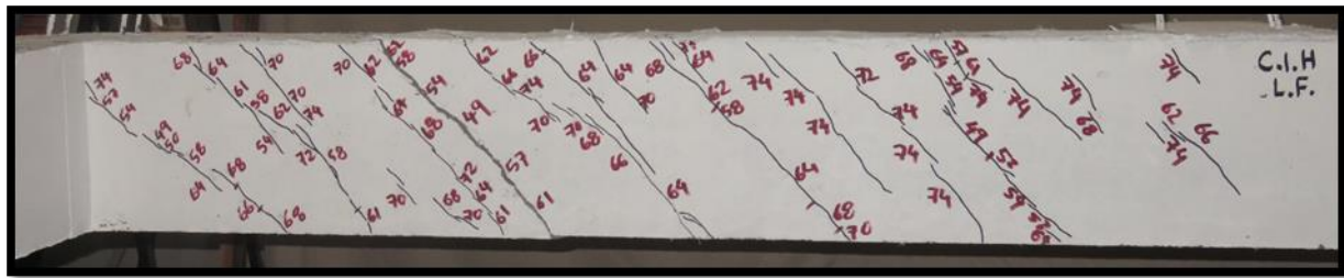
Figure 15. Crack patterns of beam C-1-H
