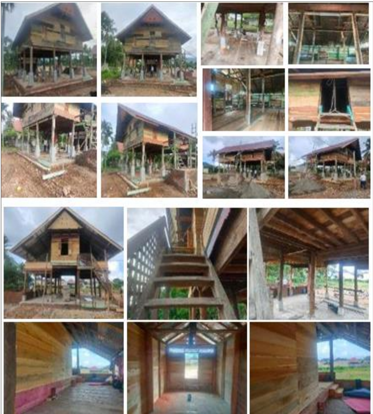
Figure 1: Reconstruction of Two Acehese Houses in Banda Aceh City. Source: Documentation, 2025
